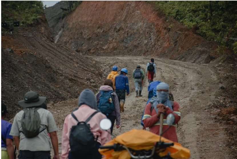
Road network between WTG 11 & 20
