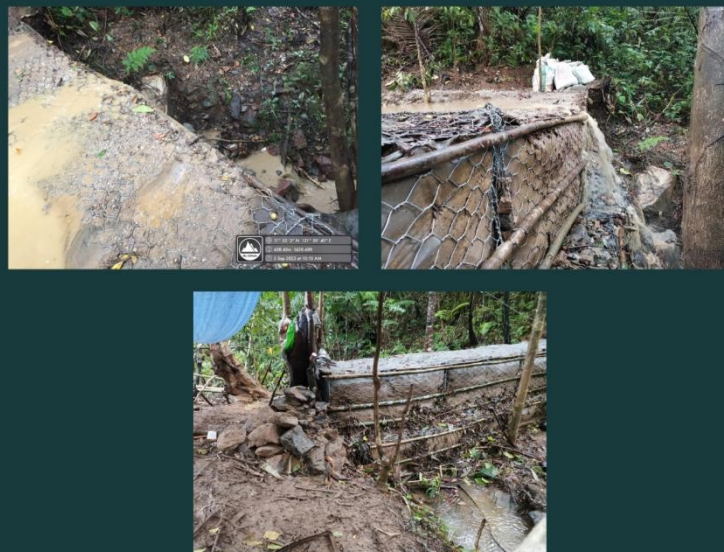
STATUS OF GABIONS
