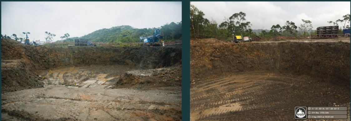
PLATFORM CONSTRUCTION (WTG20)
