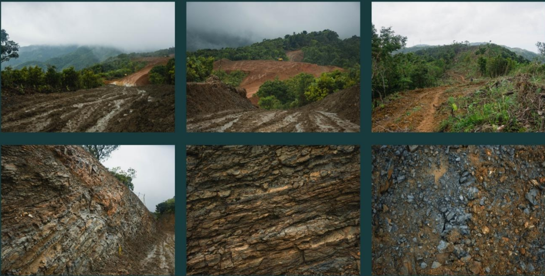
ROAD NETWORK CONSTRUCTION (WTG 20 - 25)
